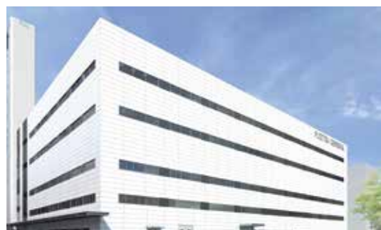
Technology Research Building (Japan)
