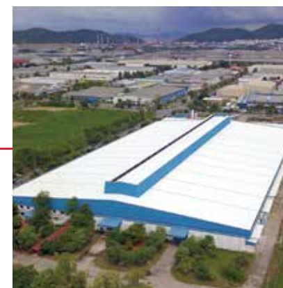
Fujitsu General (Thailand) Co., Ltd. (Thailand) FACTORY-2
