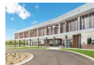
Fujitsu General (Aust.) Pty Ltd. (Australia)
