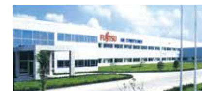
Fujitsu General (Shanghai) Co., Ltd. (China)
