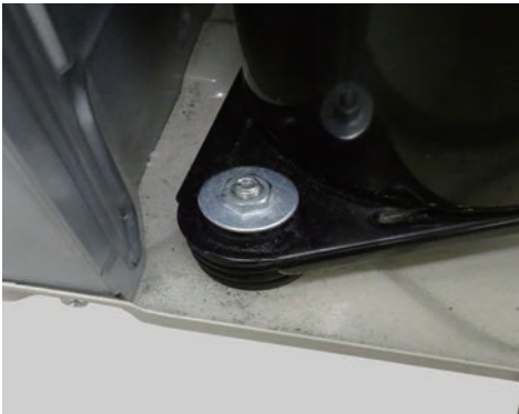
5. Remove the Compressor bolts. ( 3 places )
