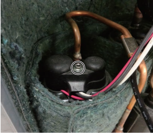
3. Remove the Hex socket screw and compressor terminal cover.
